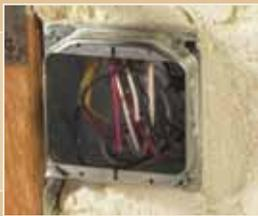
ELIMINATES GAPS AROUND ELECTRICAL OUTLETS AND CONDUIT.
